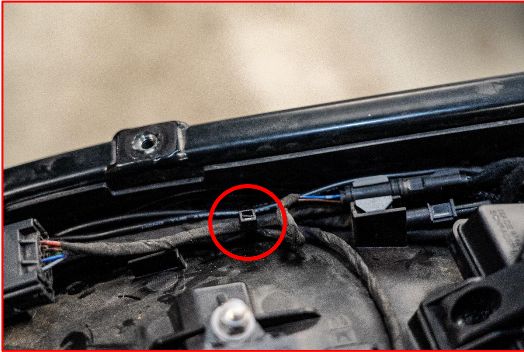
Secure the leads running to the motorcycle battery to the motorcycle wiring harness with a cable tie (circle).
